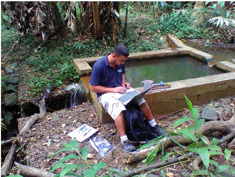
Source: Connect Saint Helena. LevelScout Data Logger Installation
